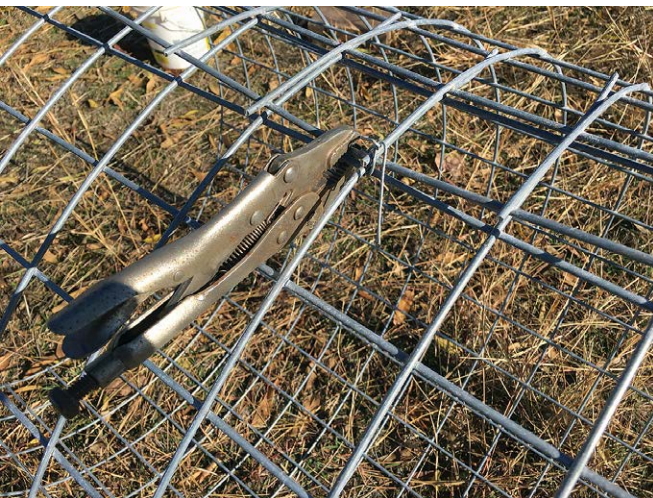
Fig 7.6: Using vice grip locking pliers to hold mesh together on a steel guard so tie wire can be fastened.
