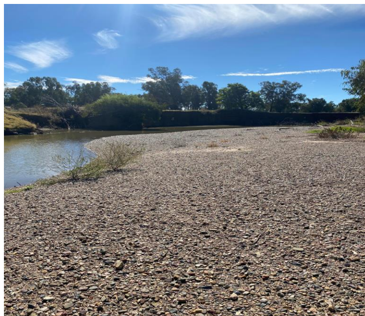
Recent flood damage to Namoi River banks.
